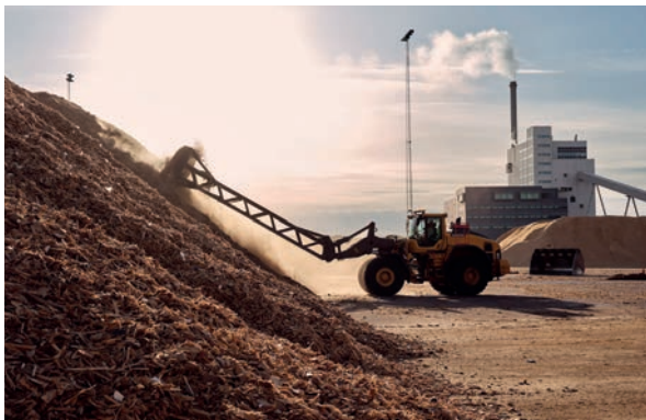
Örtoftaverket Combined Heating and Power (CHP) plant, fueled with biofuels.
