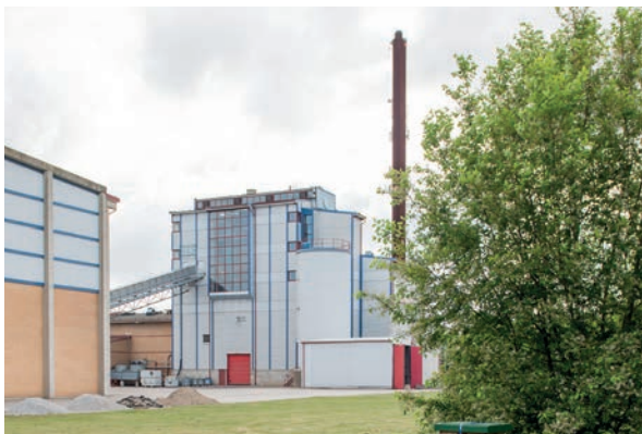
Återbruket Combined Heating and Power (CHP) plant, fueled with biofuels.
